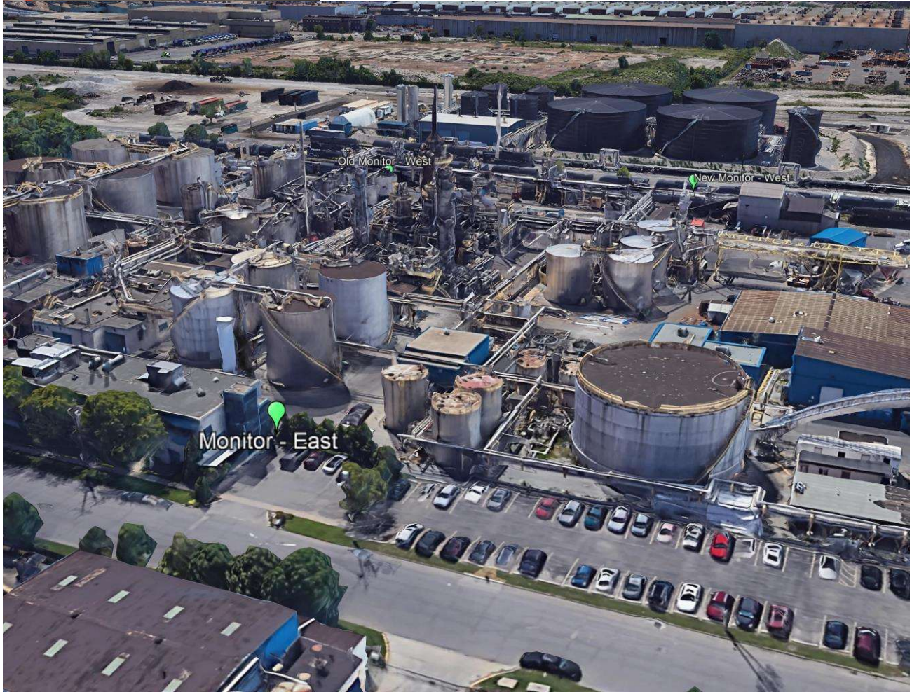
Figure A4: Aerial View 4 – East Monitoring Station
