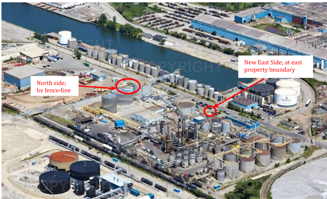
Figure 4: Monitor Locations on the North Side and East Side of the Facility
